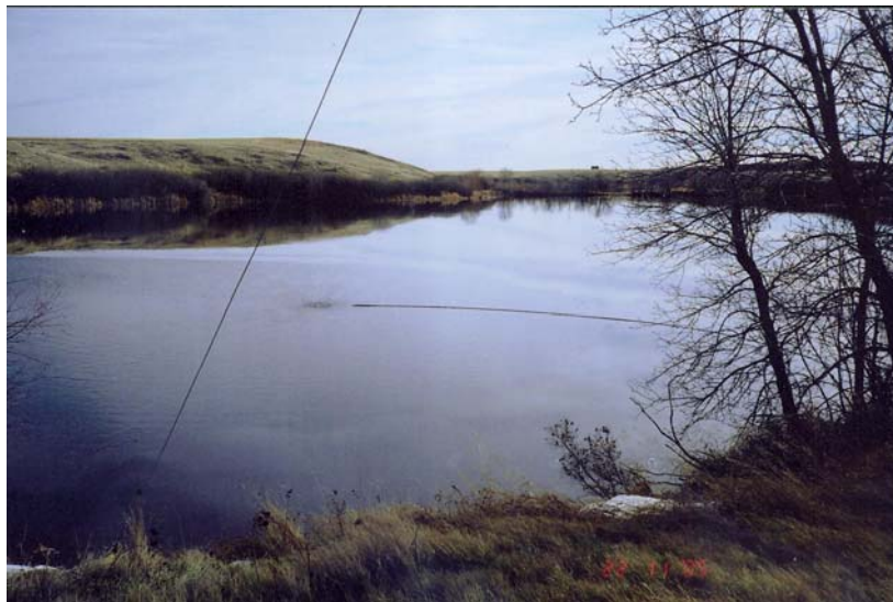
Figure A.7 Cabri's Potable Water Reservoir Nov 22, 2005 (Photo: E. Wheaton, Saskatchewan Research Council)
