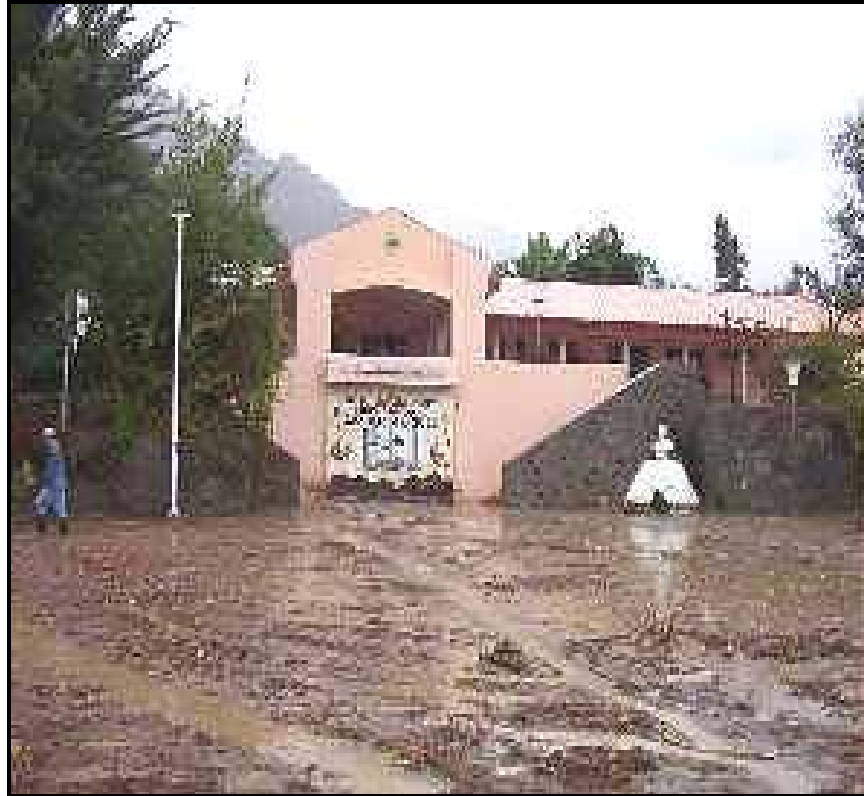
Figure 5.4. Mud flowed through the school (Zavala, H., 2004).
