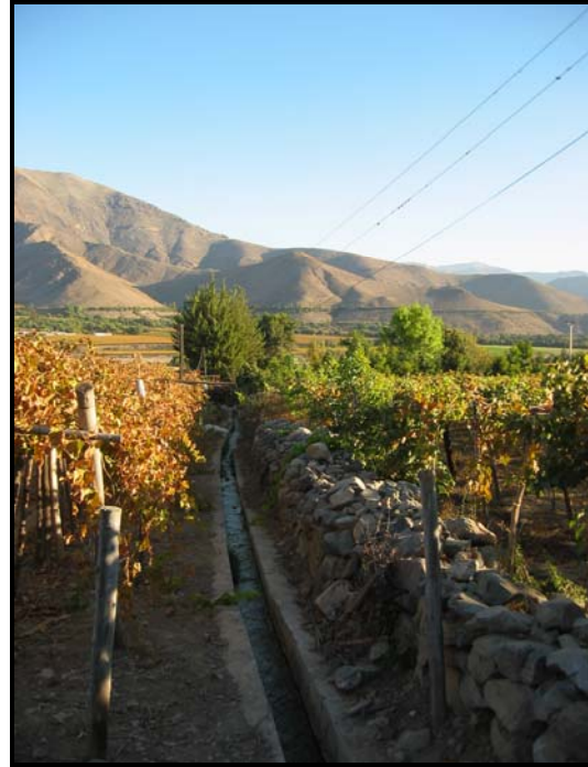
Figure 5.7. Cement lined canal in a commercial vineyard to minimize water loss.
