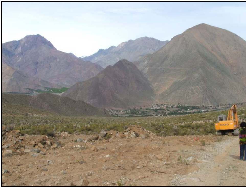
Figure 6.2. Land being leveled for commercial vineyards in Diaguitas.
