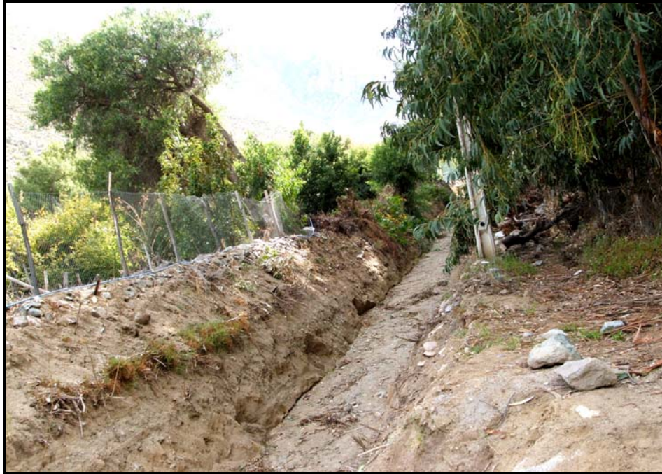
Figure 5.9. A channel constructed by the DOH to divert water and debris.
