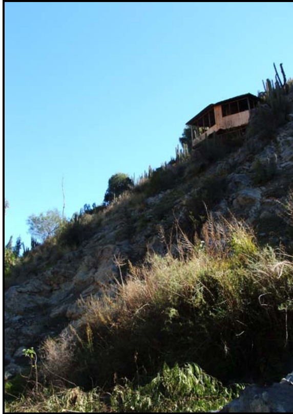
Figure 5.5. House on Mamalluca not connected to potable water system.
