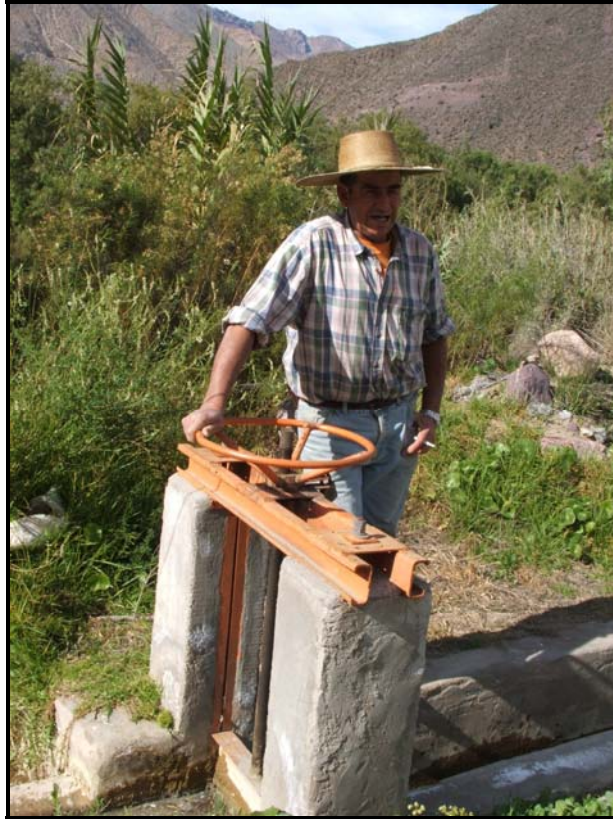
Figure 4.3. President of a canal in Diaguitas demonstrating how the water level is regulated in the canal.
